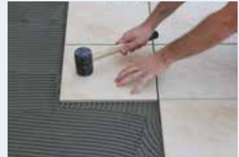
Leveling with a hammer
