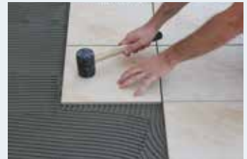
Leveling with a hammer
