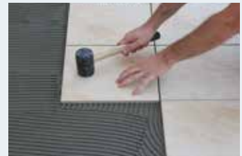
Leveling with a hammer
