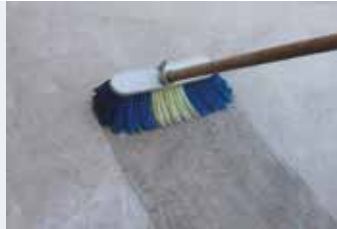
Cleaning and moisturizing the surface
