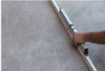
Controlling surface smoothness
