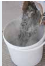
Adding mortar to the water
