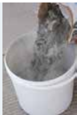
Adding mortar to the water
