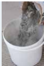
Adding mortar to the water
