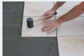
Leveling with a hammer
