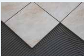
Placing the ceramic tile
