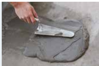
Spreading mortar through the surface with a trowel
