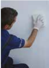
Fixing the surface of joint with a damp sponge
