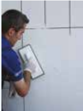
Applying grouting material on the wall
