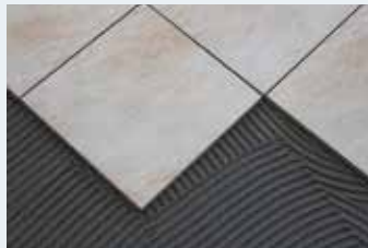
Placing the ceramic tile
