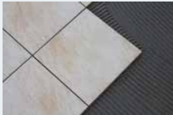
Placing the ceramic tile
