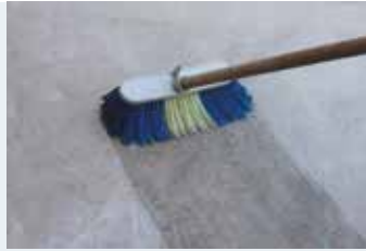
Cleaning and moisturizing the surface
