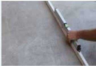
Controlling surface smoothness
