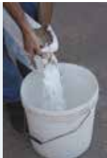
Adding mortar to the water
