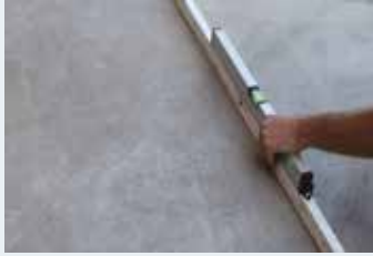
Controlling surface smoothness
