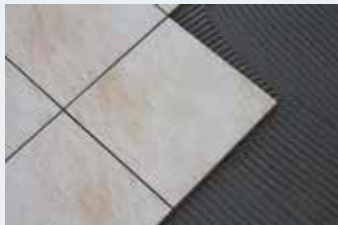
Placing the ceramic tile
