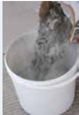
Adding mortar to the water
