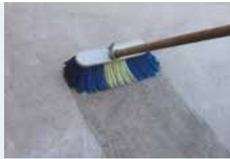
Cleaning and moisturizing the surface
