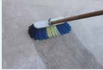
Cleaning and moisturizing the surface
