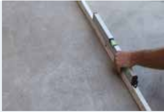
Controlling surface smoothness
